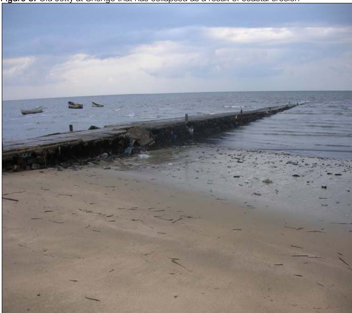
Figure 8: Old Jetty at Shenge that has collapsed as a result of coastal erosion
