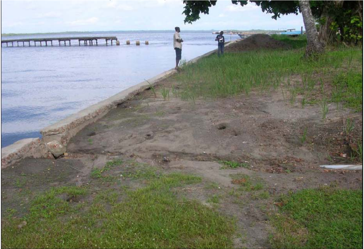
Figure 3: Part of the shoreline of Bonthe Town showing the defensive wall constructed to reduce erosion. Now the high tide water goes over this coastal defense barrier.
