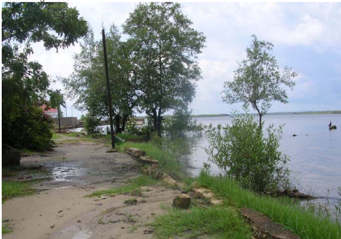
Figure 15: Defensive wall build in the 50s no longer protect the coastline as this wall is under water at high tides
