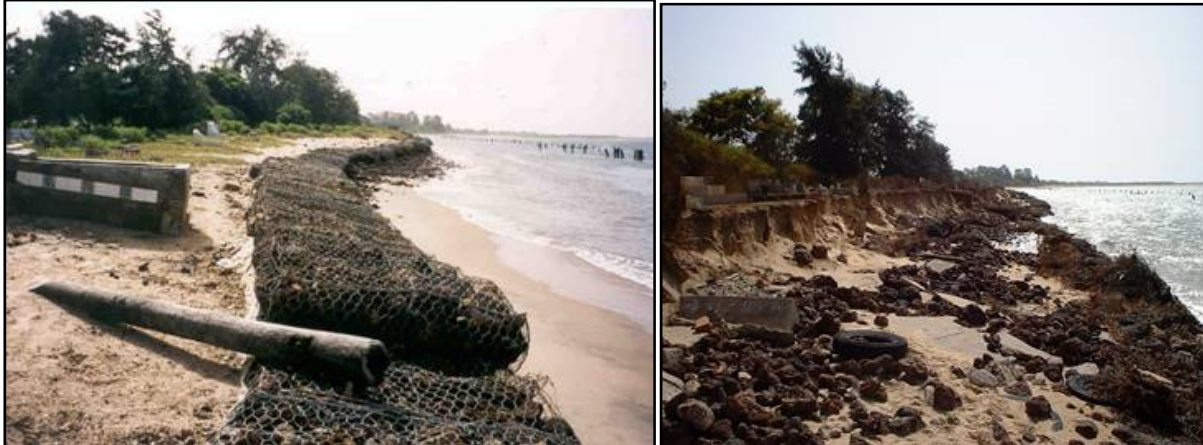
Photos 15&16 : Erosion at Muslim Cemetery and Temporal measures implemented
